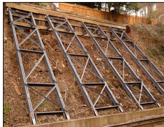
(After: None corrosive FRP shoring installed to support bank)
