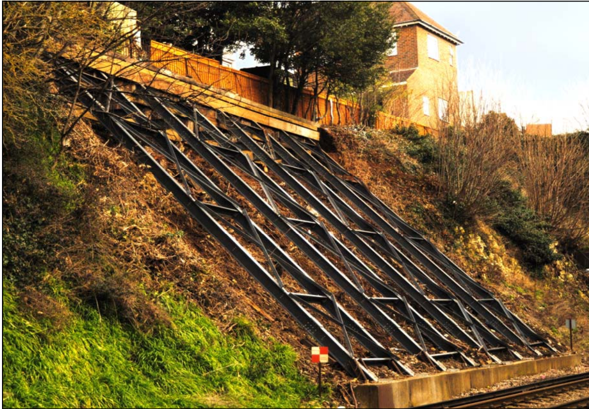
(FRP shoring installed)
