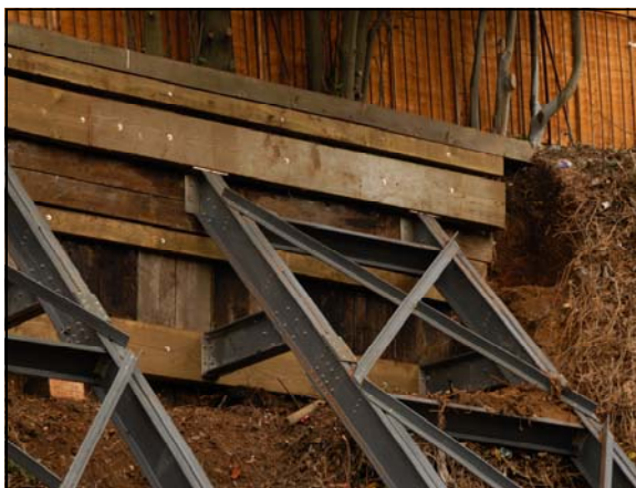
(FRP shoring bolted into position)
