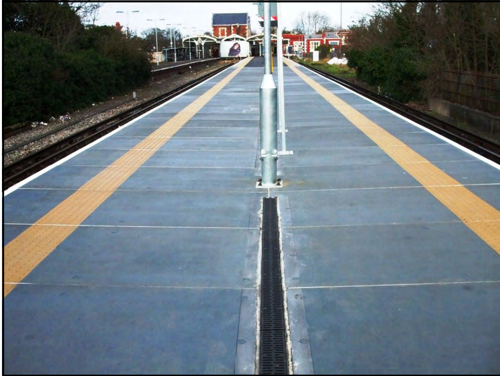
(FRP platform fully installed at Hampton Court Railway Station)
