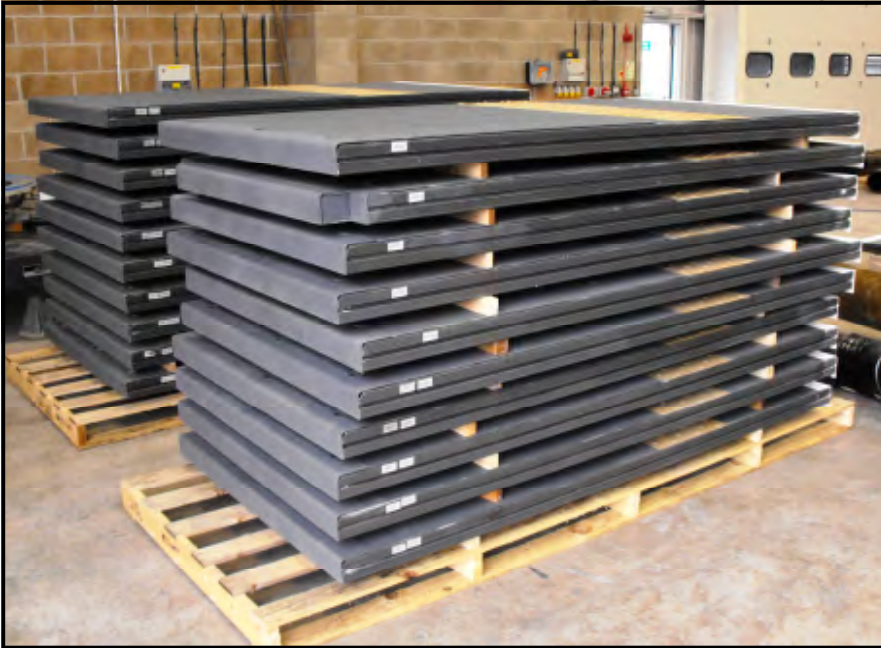
(20 No. of the 158 No. FRP deck panels stacked ready for delivery & installation)
