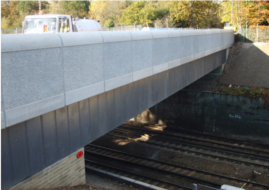
(Chislehurst road bridge FRP enclosure fully installed)
