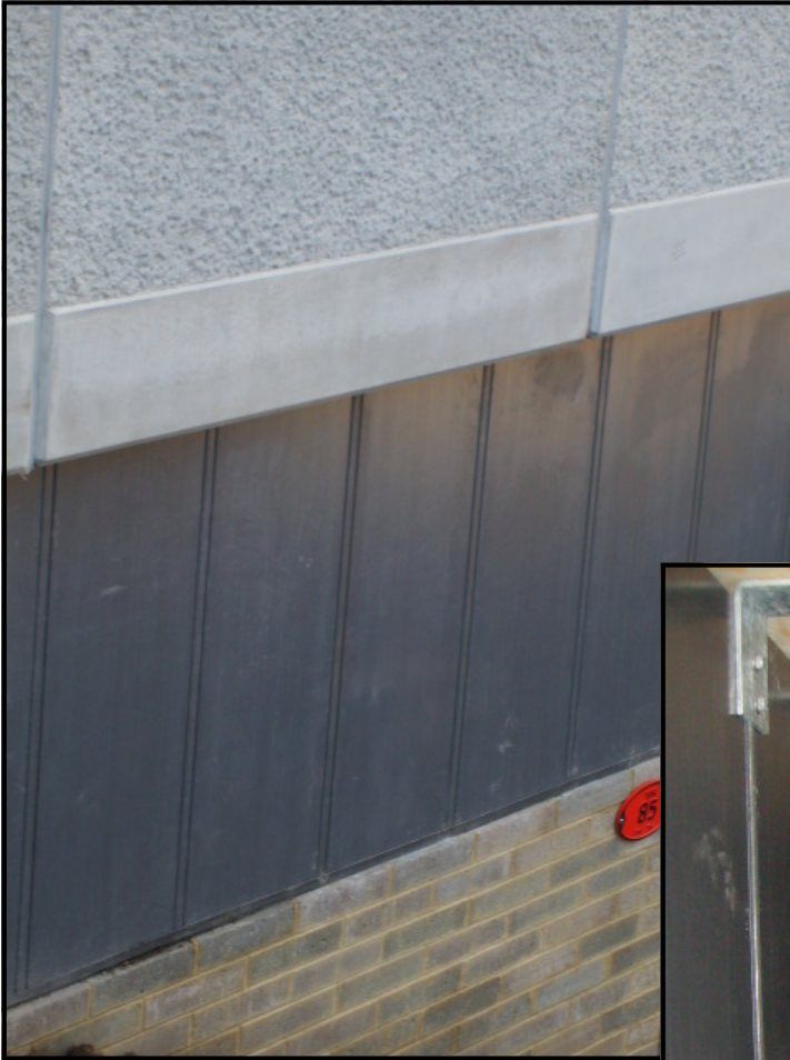
(Detail of FRP enclosure panels installed on Chislehurst road bridge)
