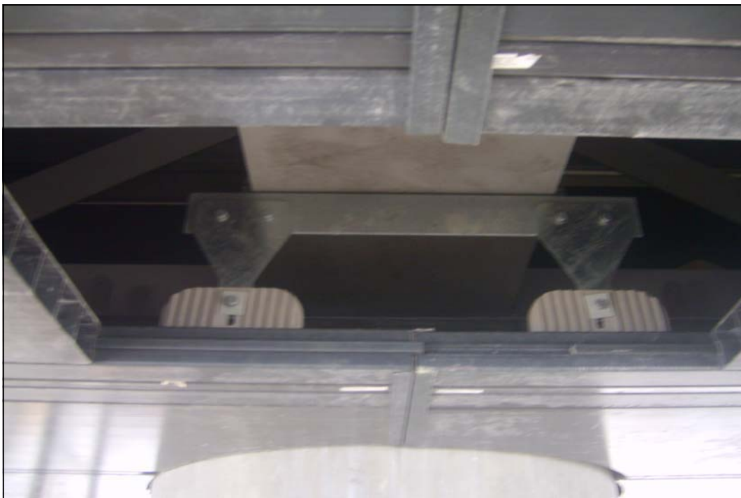
(Pipex px ® hanger system: connectors securing composolite panels to bridge steelwork)
