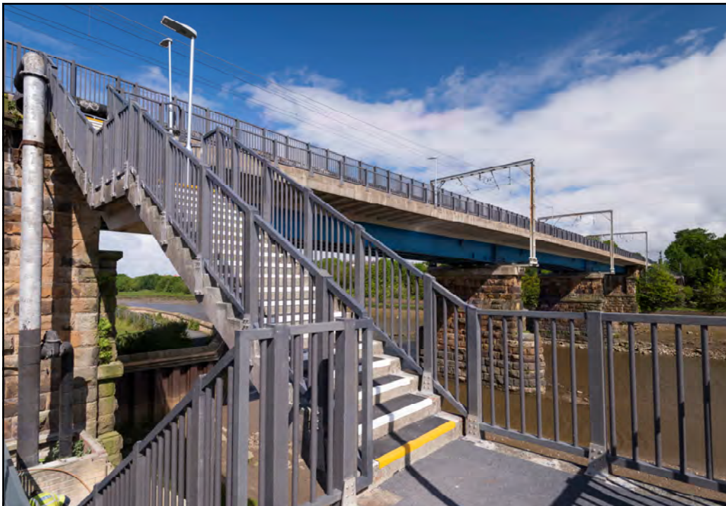
(Pipex px ® FRP handrails installed)
