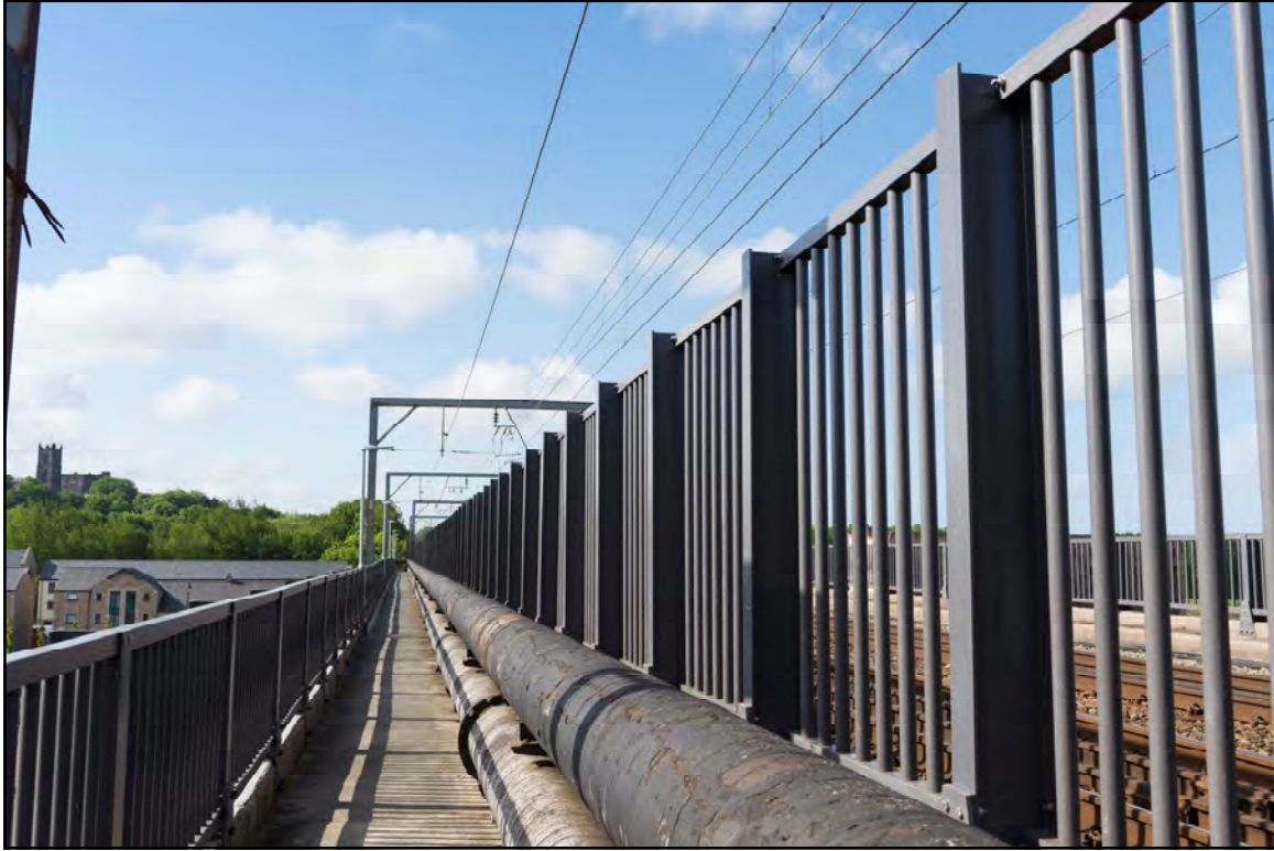
(Pipex px ® FRP Parapet Fencing installed on Carlisle bridge)
