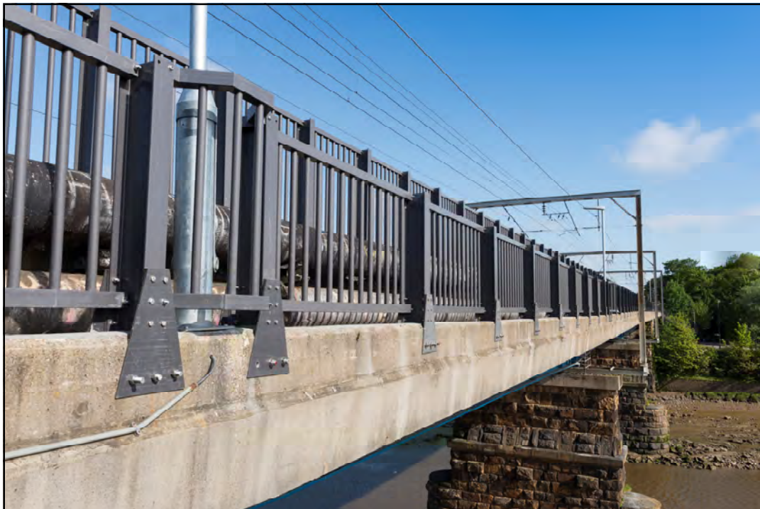
(Pipex px ® FRP Parapet Fencing installed)
