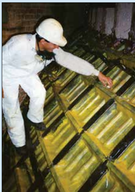
FIGURE J.9-1: Stiffeners placed within a flat FRP panel
