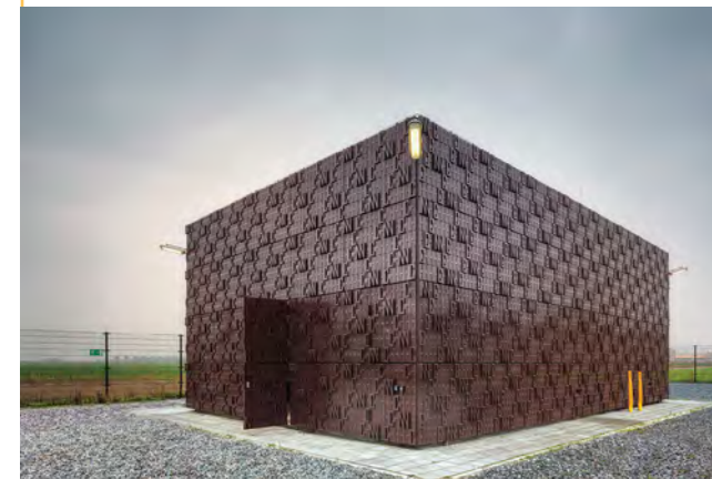
Figure 18: A bio-based façade made from hemp and part-bio resin (Gas receiving station clad in biocomposite panels. Location: Agro and Food Cluster, New Prinsenland, Netherlands. Architect: Marco Vermeulen. Manufacture: NPSP Composites, Haarlem. Photo ©Robert Tilleman).
