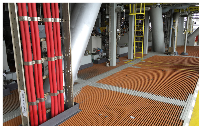
Phenolic grating installed on an offshore platform in the North Sea. Photo courtesy of NOV Fiber Glass Systems
