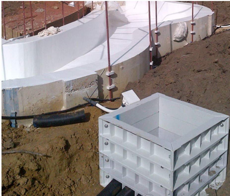
Cubis Systems carry out EPDs for many of their products, including this GFRP RapidSTACK™ chamber. Photo courtesy of Cubis Systems.
