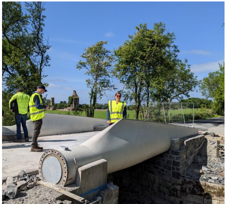
BladeBridge installed on the Midleton Youghal Greenway, Cork County. Photo courtesy of the Re-Wind Network
