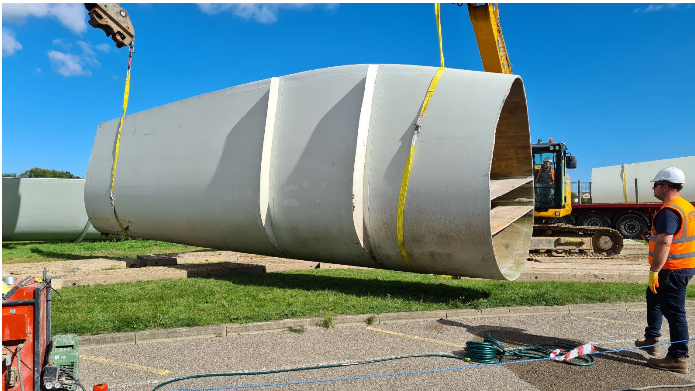
For large items like wind turbine blades, downsizing is a challenge before any recycling route can be pursued. Photo courtesy of Reblade
